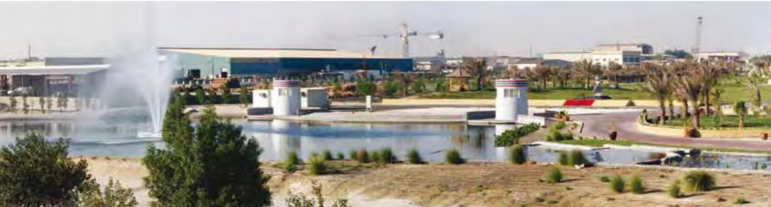
Blow-down water from Casthouse Alba Oasis lake
