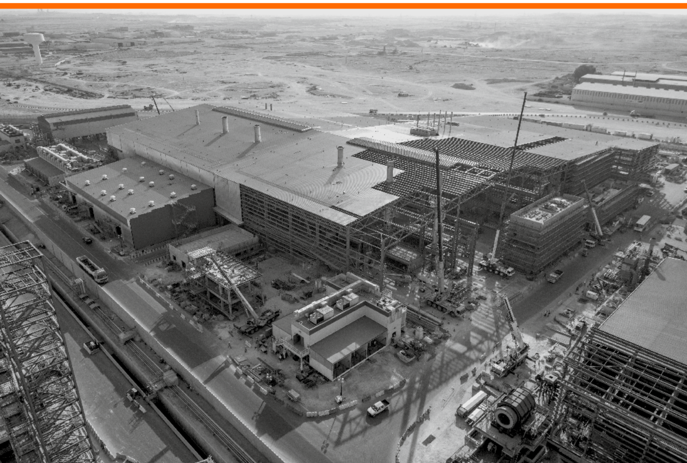
Aerial View of Line 6 Expansion Project: Casthouse Area
