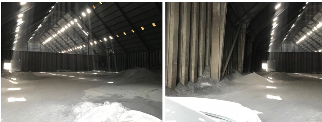
Figure 2.7 Existing Coke Storage Shed
