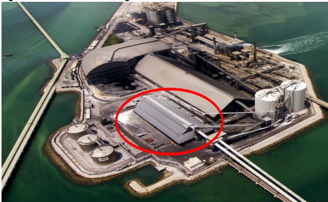
Figure 2.8 Location of Storage Silos
