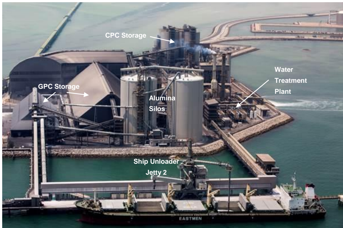
Aerial shot looking westwards of vacuum unloader on Jetty 2
