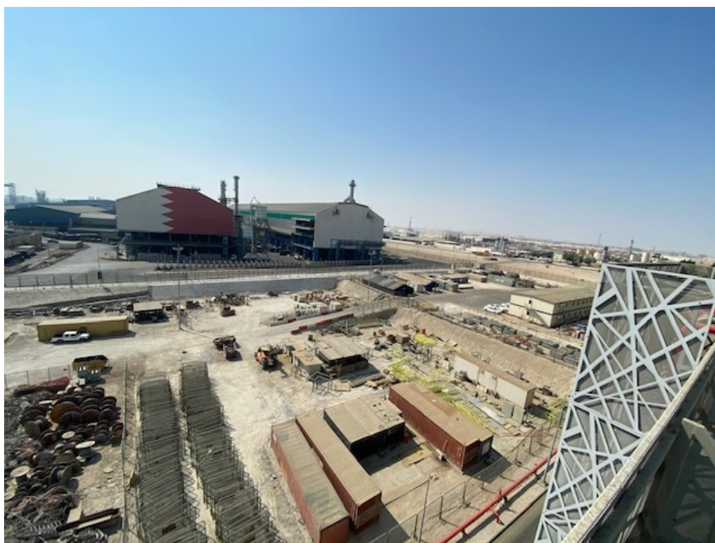
Figure 14-1 Overview of the Project Site
