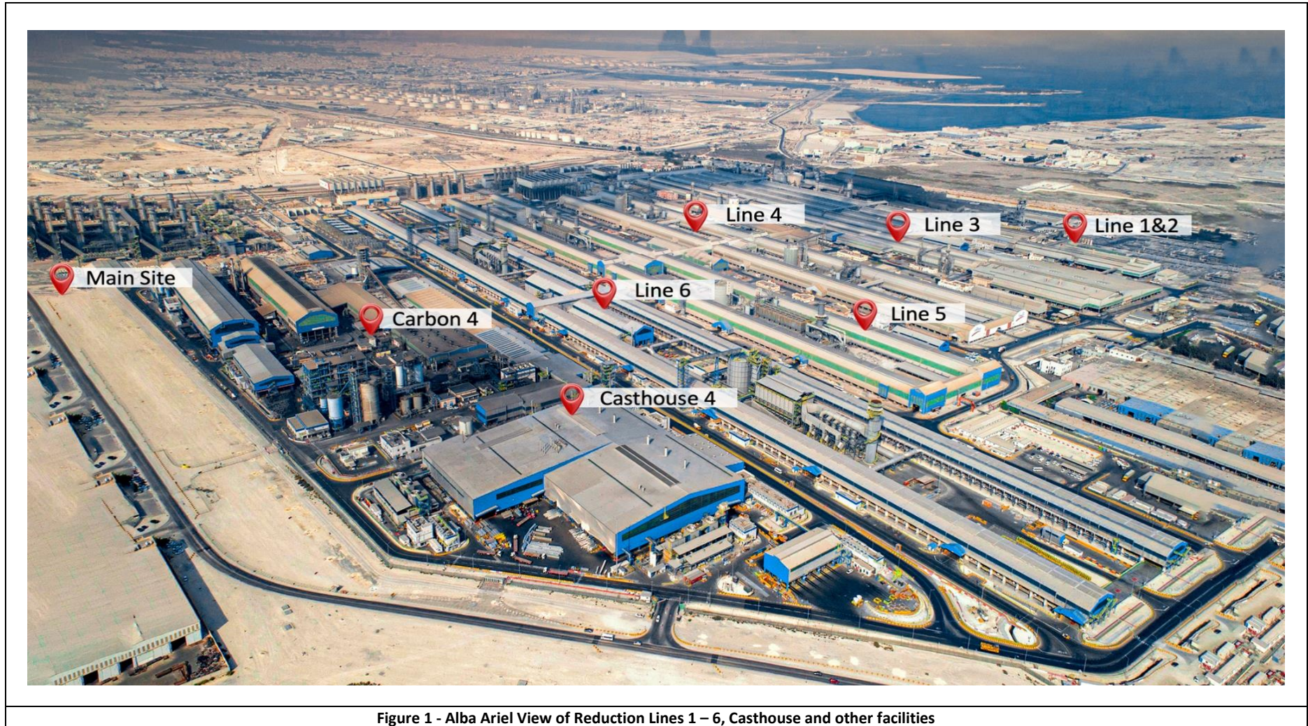
Figure 1 - Alba Ariel View of Reduction Lines 1 – 6, Casthouse and other facilities
