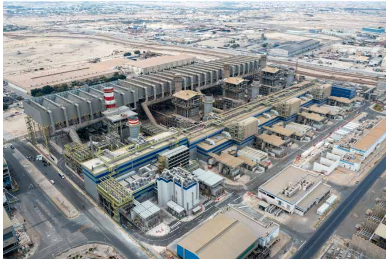
Aerial view of Alba's Power Station 5 Block 4
