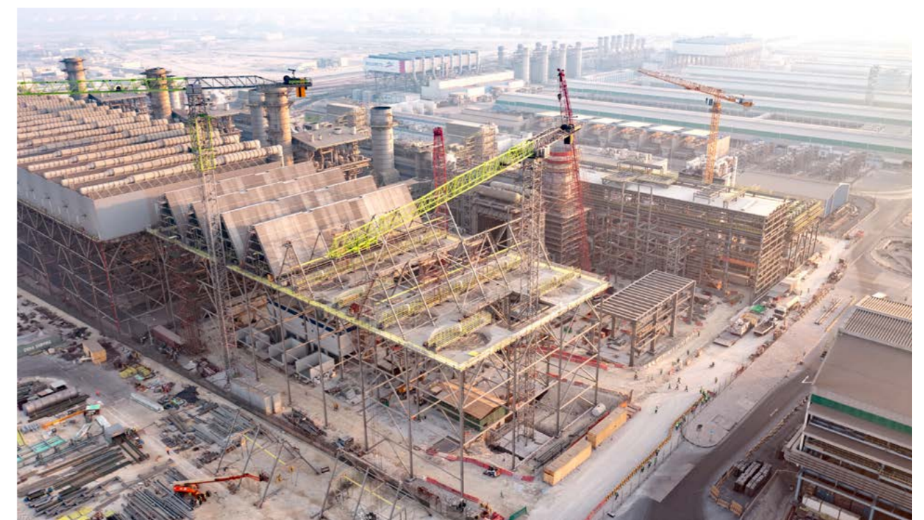
Aerial View of PS5 Block4 Project
