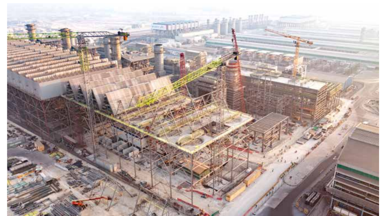
Aerial View of PS5 Block4 Project
