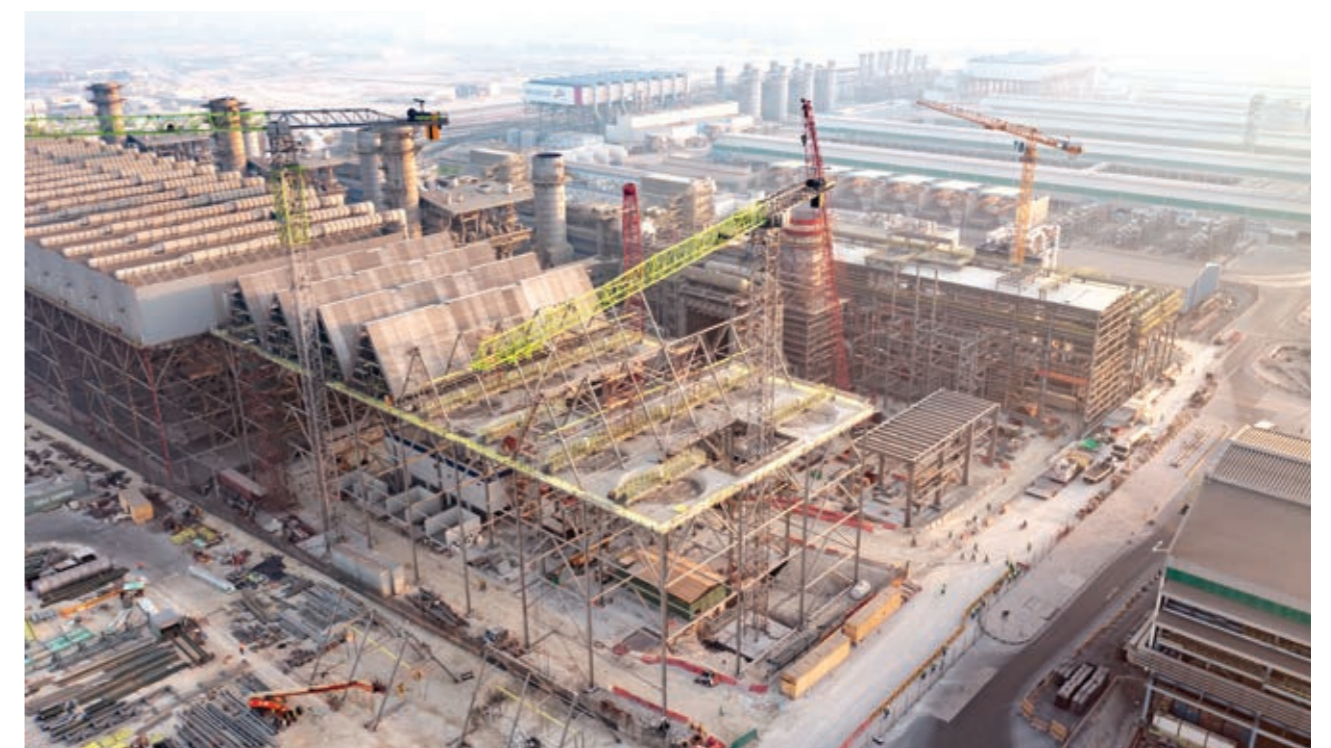
Aerial View of PS5 Block4 Project
