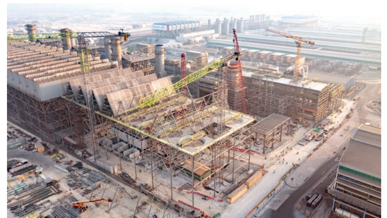
Aerial View of PS5 Block4 Project
